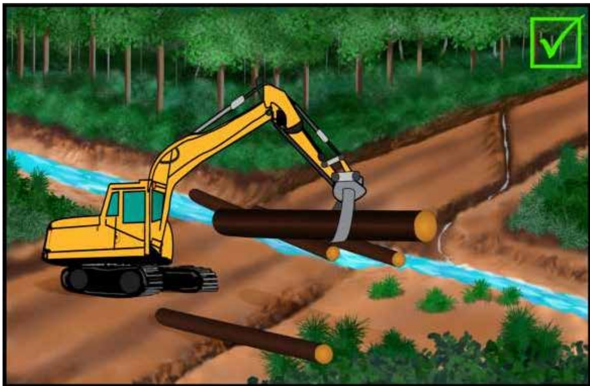
Figure 80: Remove logs from stream crossings used during skidding
